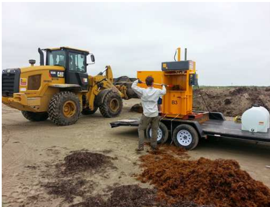
Figure 2.4: Photo of dune construction and seabaling operations. The dune was constructed using heavy front-loaders.
