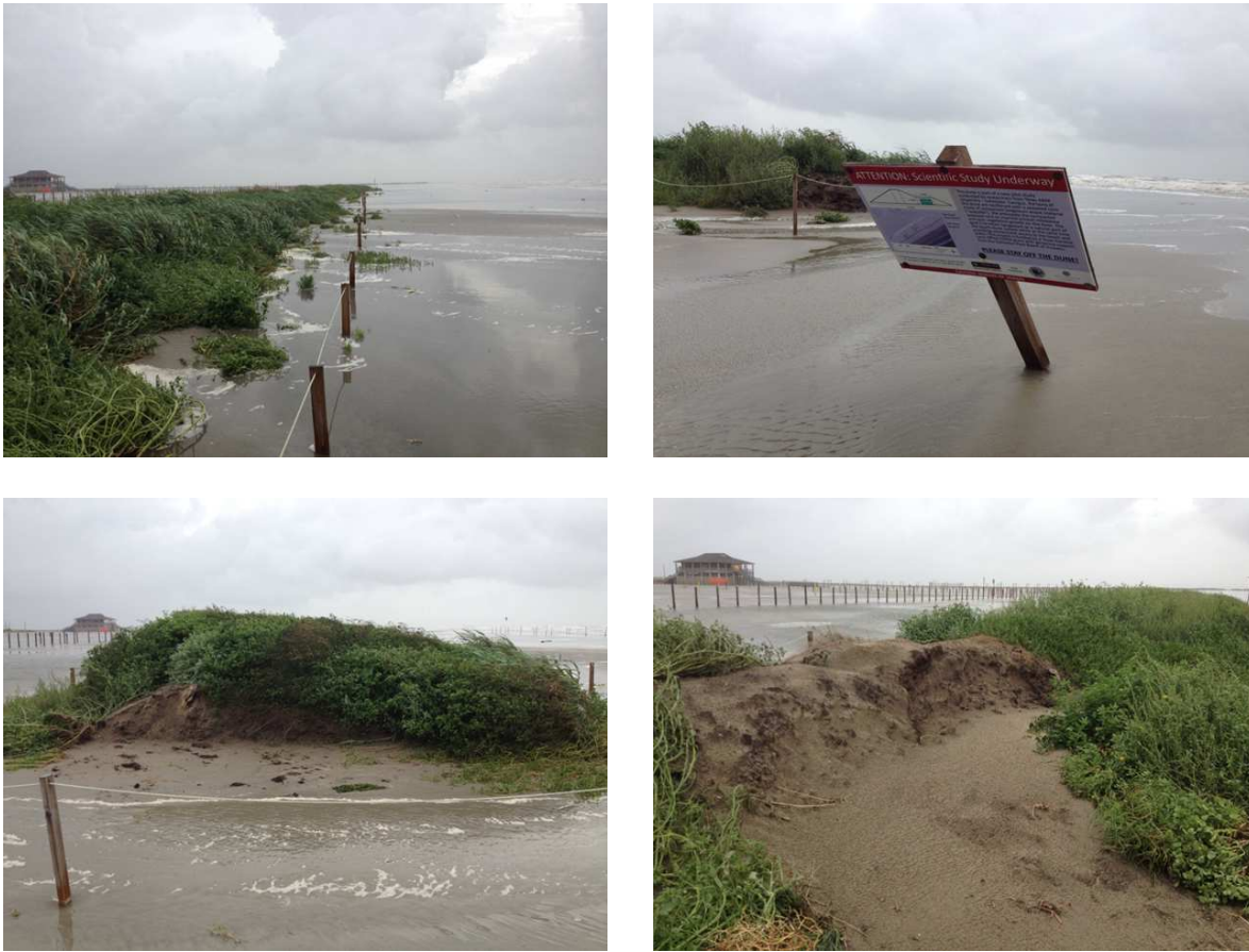
Figure 4.2: Photos of the prototype dune taken one day after tropical storm “Bill” hit the Texas coast on June 16th, 2015. Top left: Dune segment 1 performed extremely well since the combination of planted vegetation and seabales had created a strong berm to withstand the wave attack during the storm. Top right: The tilted project sign in a gap between two dune segments illustrates the wind and water forces acting on the area during Bill. Bottom left: Strong currents flowed through the planned gaps between dune segments eroding some of the edge material. Bottom right: Dune segment 4 without seabales and initial vegetation showed the most significant erosion and dune scarp retreat caused by Bill.
