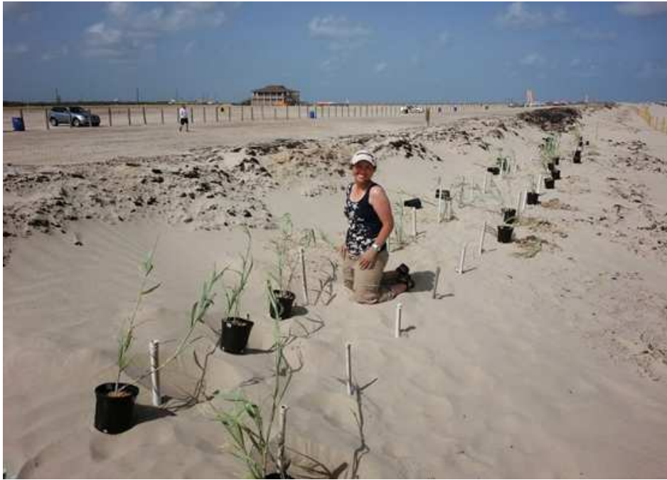
Figure 2.7: Photo of initial vegetation planting. Panicum amarum was planted on the berm of dune segments 1 and 2 after initial dune construction was completed.
