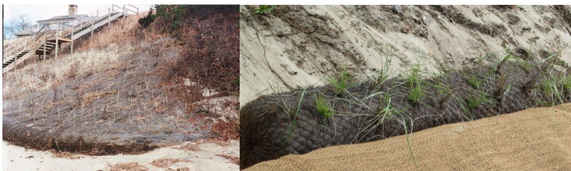
Figure 37. Photos of bio-thatching (left) and fiber coir roll (right) applications for coastal dune stabilization projects (source: Massachusetts Office of Coastal Zone Management).
