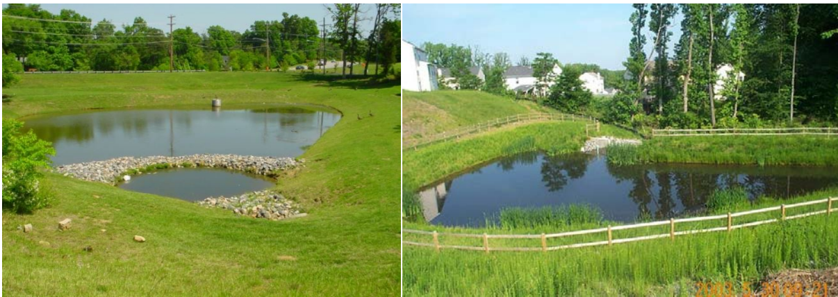
Figure 21. Photos of retention basins installed alongside a road (left, source: City of High Point, NC) and alongside a residential area (right, source: Charles County government, MD).
