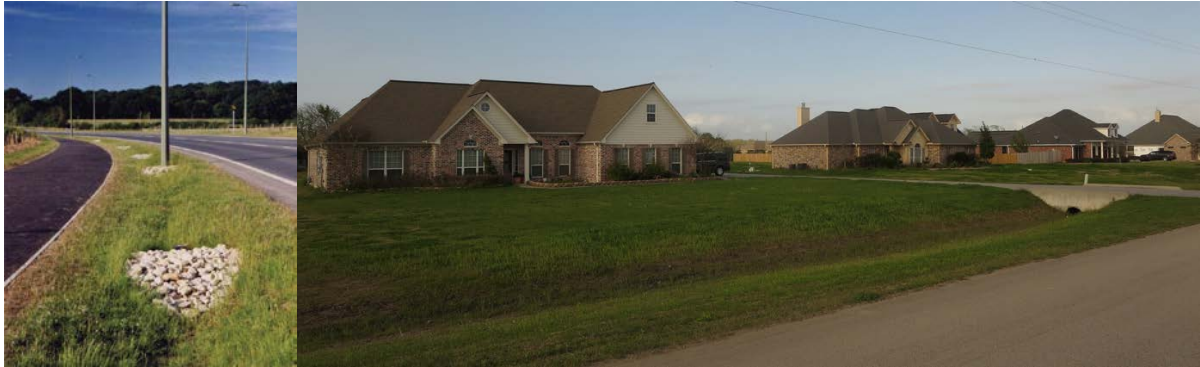
Figure 29. Photos of dry swales in urban settings. A shallow vegetated swale with check-dams alongside a distributor (pervious) road (left, source: Cambridge City Council) and a typical application in a residential neighborhood in Chambers County, Texas. (Source: Barrett et al., 2014).
