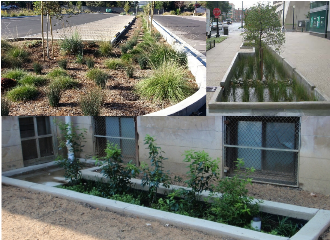
Figure 27. Photos of examples of bioretention in a parking lot (top left; source: Casey Patterson, Central Coast Low Impact Development Initiative), with drop curbs in a street setting (top right; source: National Association of City Transportation Officials), and as flow-through stormwater planter in a residential setting (bottom; source: Philadelphia Water Department).
