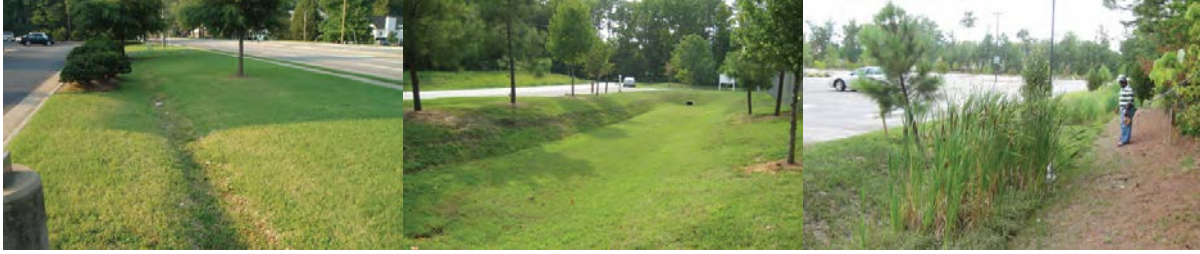
Figure 28. Photos of vegetated swale design options. Grass channel, dry swale, and wet swale (from left to right) alongside roadways and parking lots (Source: Ellis et al., 2014).
