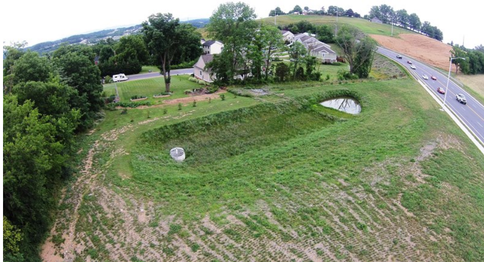
Figure 18. Photo showing an example of an extended detention basin incorporating a micropool and vegetation planting. (Source: http://www.matternandcraig.com ).
