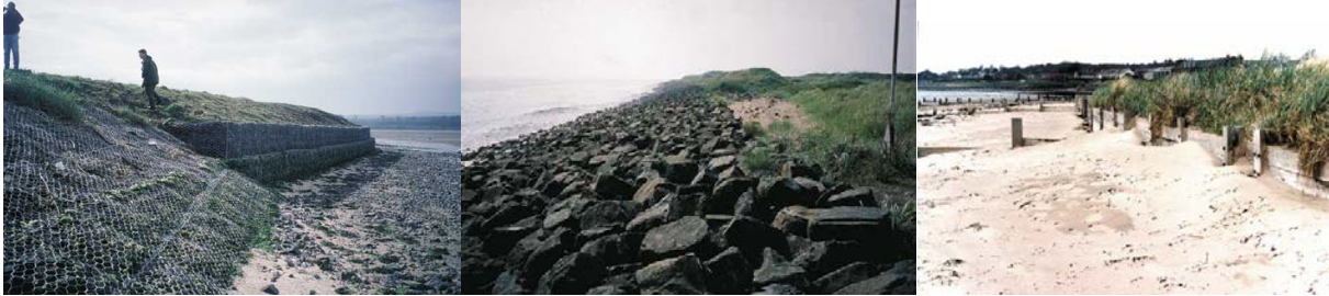
Figure 34 Photos of revetment variations for coastal dune protection. Shown are gabion mattresses and gabion walls (left), a rock armor revetment (center), and timber breastwork (right) in coastal environments (source: Scottish Natural Heritage, 2000).
